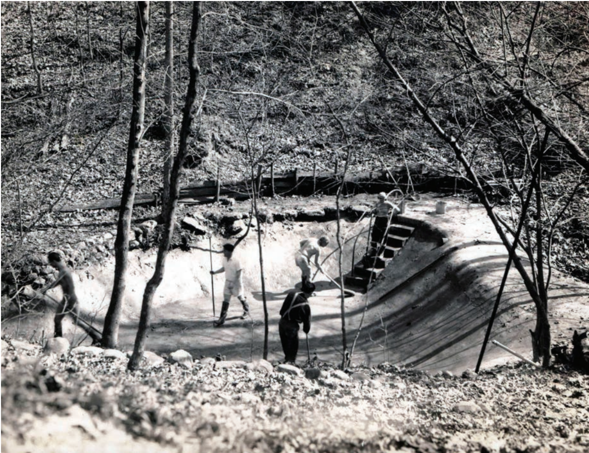
Construction of Frog Pond. nd. Credit: Alice Ferguson Foundation
